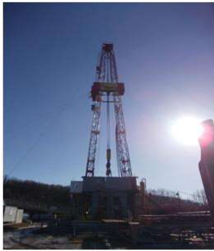
Figure 3. F320-3DH drilling rig
