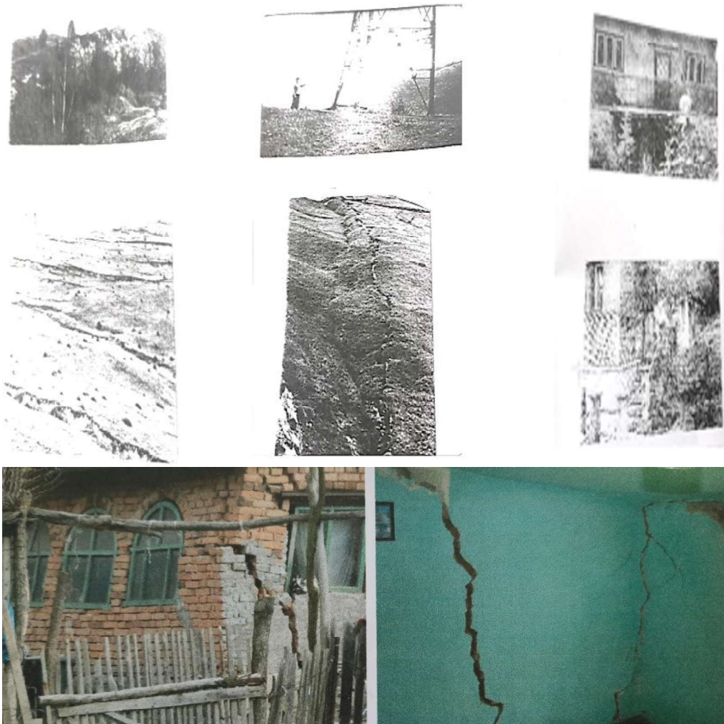
Figure 9. Subsidence phenomena in Lonea mine
