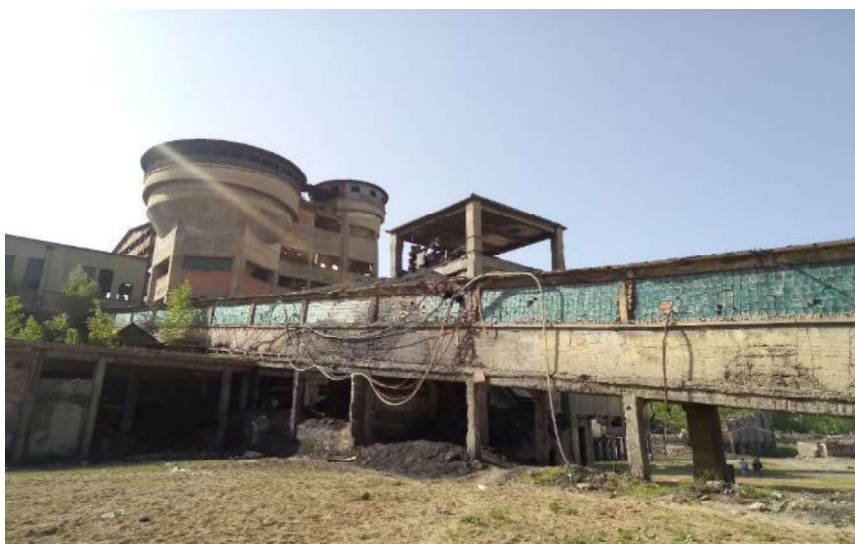
Figure 12. Overview of the old Preparation [2]
